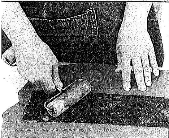
Figure 4 Press tar paper into place and lightly roll to secure it.
